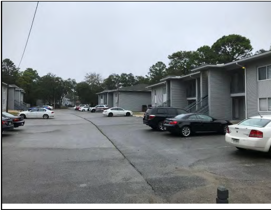
View of typical Raider Housing Building and Site Improvements
