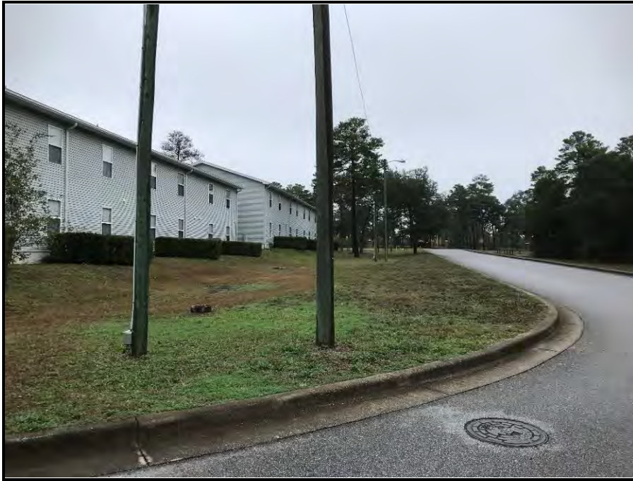
College Apartments - View of Rear / East Elevations from Garden Lane, Facing North
