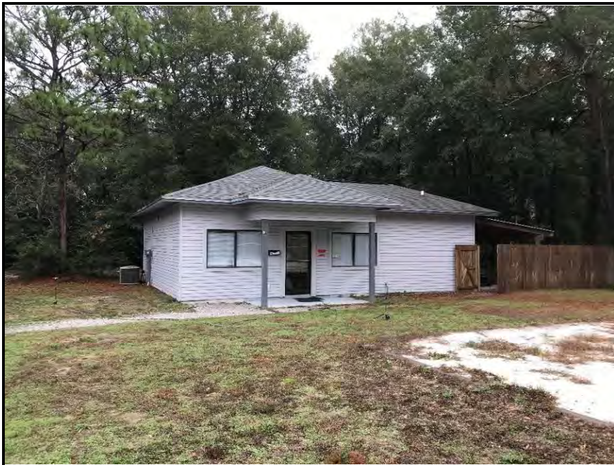
View of Laundry/Office/Maintenance Building
