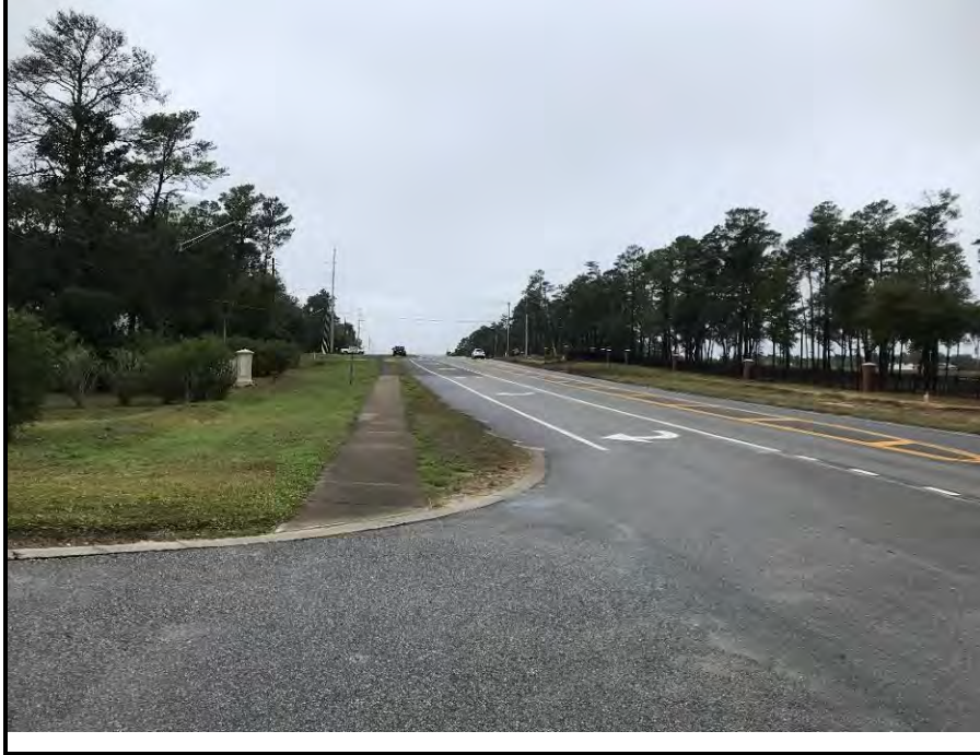
View Facing West along College Boulevard East, Subject on Left
