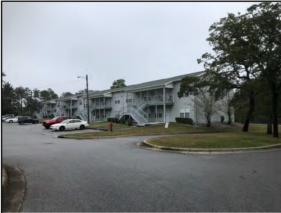
Front View of College Apartments Rental Housing
