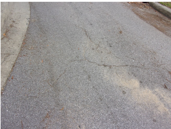
Photo Exhibit No. 63 Alligator cracking within main drive lane.
