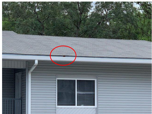
Photo Exhibit No. 18 Corrosion on metal roofing components on the student housing roof.
