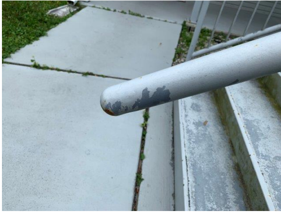
Photo Exhibit No. 25 Coating on railing needs to be touched up.
