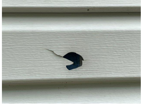
Photo Exhibit No. 22 Large hole in siding, no WRB visible beneath.
