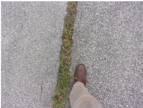
Photo Exhibit No. 57 Large cracking in asphalt that has become overgrown.
