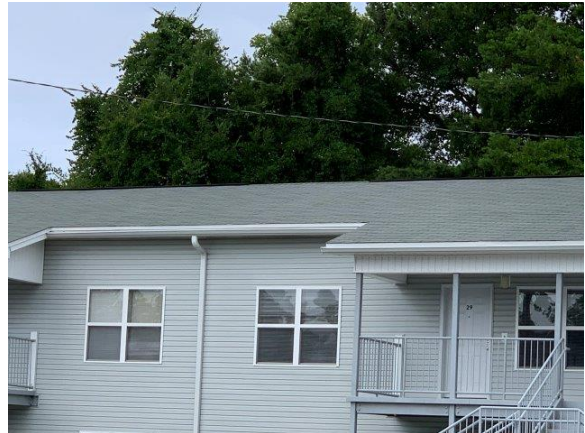
Photo Exhibit No. 11 Apartment roof shingles in fair condition.
