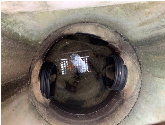
Photo Exhibit No. 56 Large amount of sand in catch basin and visible within pipe as well.
