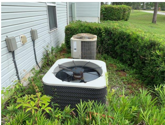
Photo Exhibit No. 45 Exterior units appear to be in good condition, minor housing corrosion observed.
