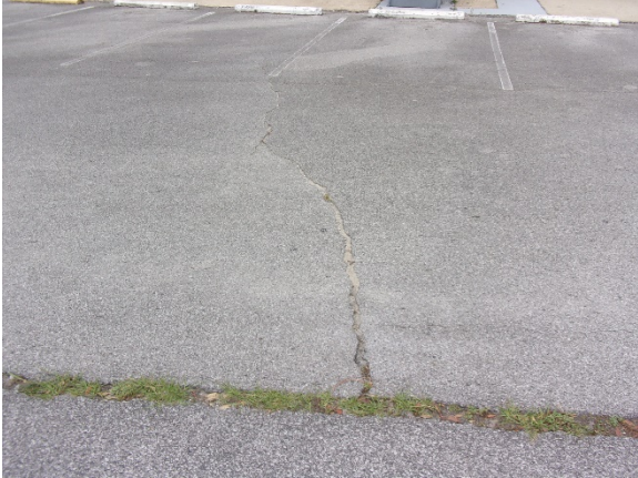
Photo Exhibit No. 61 Large crack extending length of parking lot.
