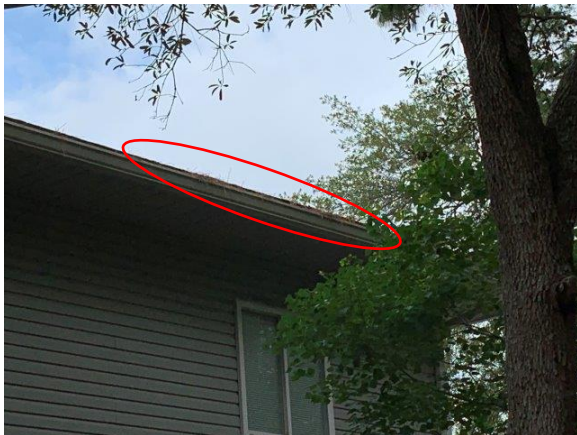
Photo Exhibit No. 14 Heavy buildup of debris in gutter on student housing building.
