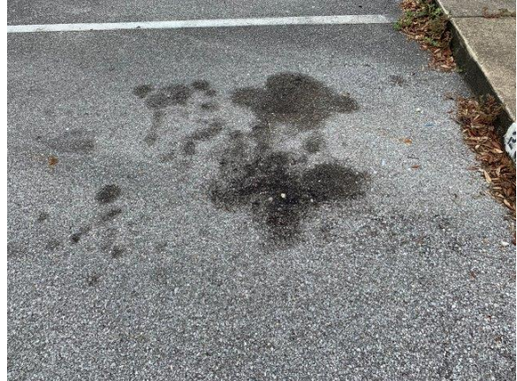
Photo Exhibit No. 64 Vehicle oils/liquids cause pre-mature failure of asphalt bitumen.
