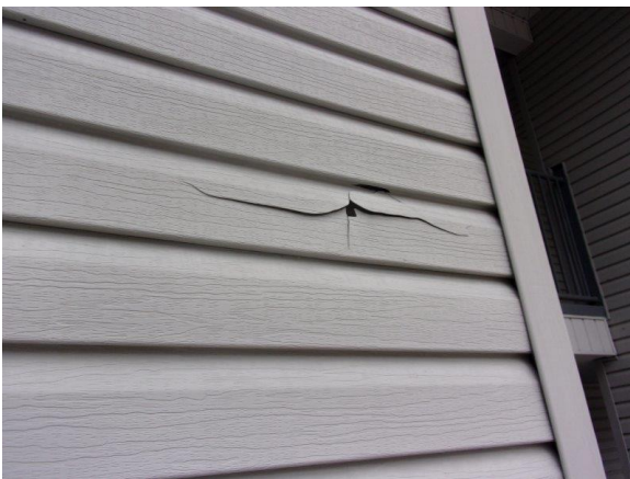
Photo Exhibit No. 21 Large crack in siding.
