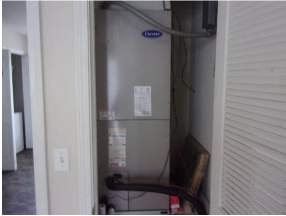
Photo Exhibit No. 43 Interior Carrier air handling unit appears to be working well.
