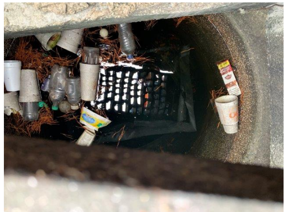
Photo Exhibit No. 54 Large amount of debris in catch basin.
