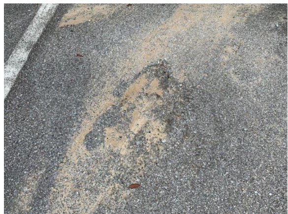
Photo Exhibit No. 66 Loss of fines and exposed aggregate.
