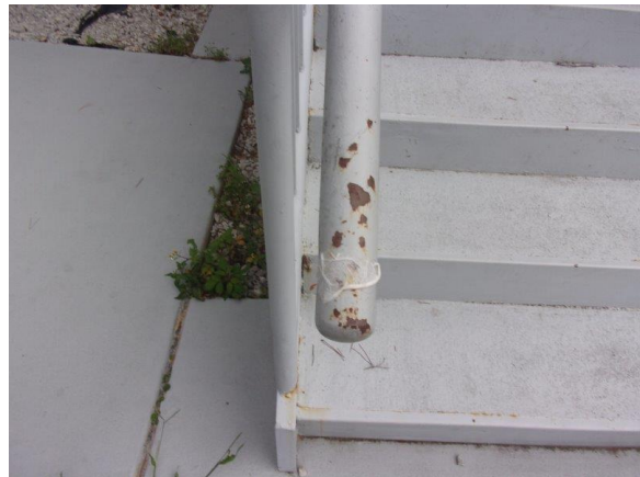
Photo Exhibit No. 29 Corrosion and paint failure on railing.
