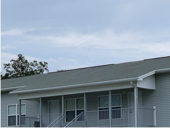
Photo Exhibit No. 7 Asphalt shingle roof on apartment building in fair condition.
