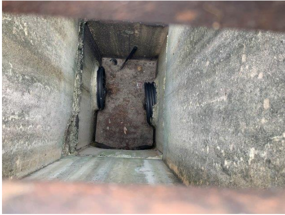
Photo Exhibit No. 55 Large amount of sand in catch basin.
