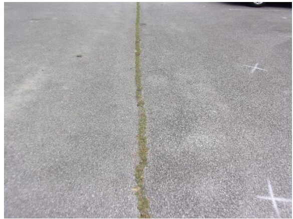
Photo Exhibit No. 59 Large crack runs entire length of parking lot in front of student housing.
