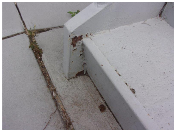
Photo Exhibit No. 30 Corrosion and coating failure on stair riser.
