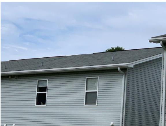
Photo Exhibit No. 9 Asphalt shingle roofing in fair condition at apartment building.
