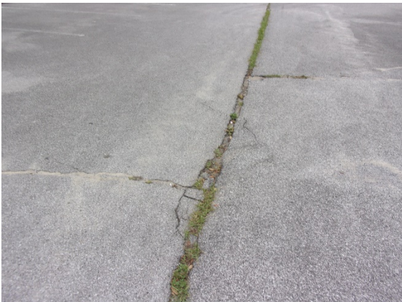
Photo Exhibit No. 62 Large crack runs entire length of parking lot Infront of student housing.
