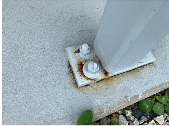
Photo Exhibit No. 28 Corrosion and minor paint failure on metal landing post.
