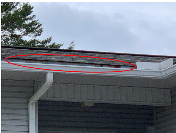
Photo Exhibit No. 15 Large amount of corrosion on shingle starter at student housing roof.
