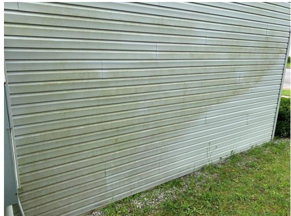
Photo Exhibit No. 23 Large area of staining on siding.
