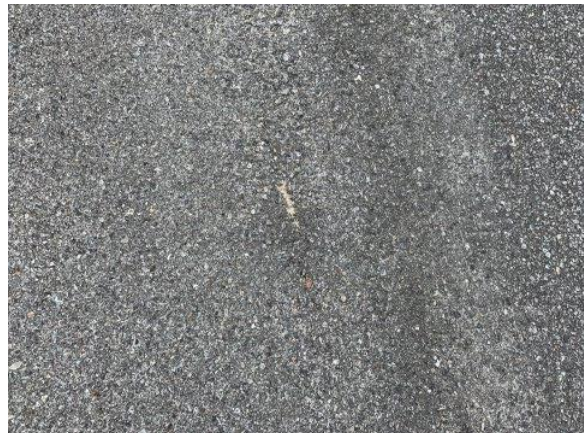
Photo Exhibit No. 65 Loss of fines and exposed aggregate.
