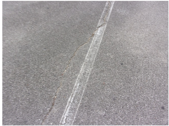
Photo Exhibit No. 60 Large crack extending from perimeter into field of parking lot.
