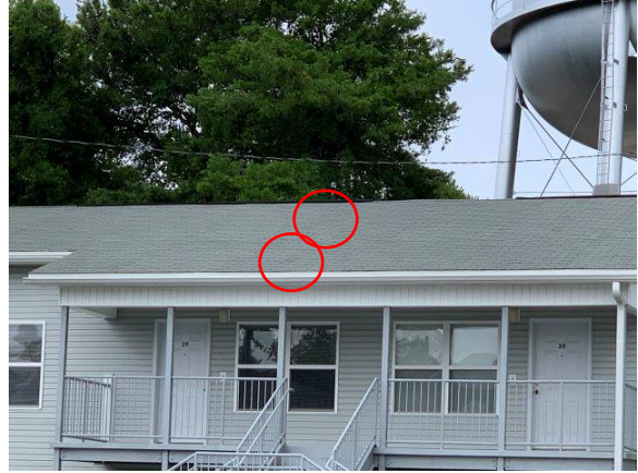
Photo Exhibit No. 10 Minor granule loss on asphalt shingles of apartment building.
