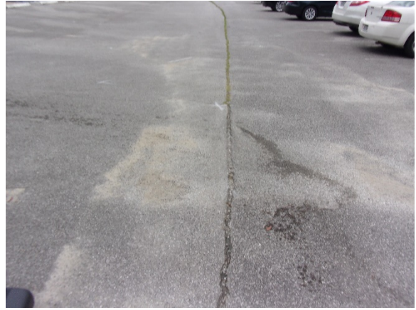
Photo Exhibit No. 58 Large crack runs entire length of parking lot in front of student housing.
