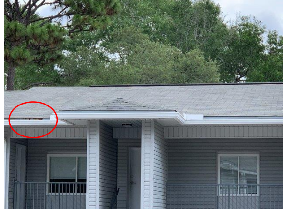
Photo Exhibit No. 16 Shingle deterioration and corrosion present on student housing roof.
