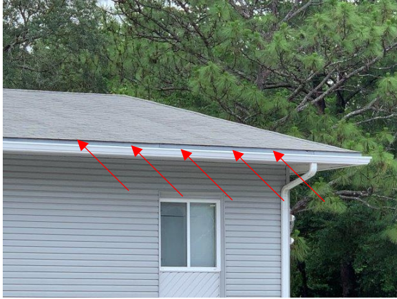
Photo Exhibit No. 13 Truss lines visible through asphalt shingles at student housing.
