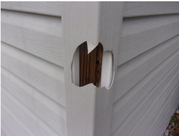
Photo Exhibit No. 20 Wood sheathing is visible beneath siding. No WRB present.
