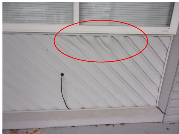
Photo Exhibit No. 24 Siding beneath this window was poorly installed.
