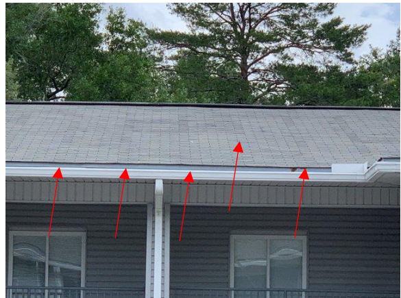
Photo Exhibit No. 17 Corrosion on metal components as well as truss lines visible through shingles.
