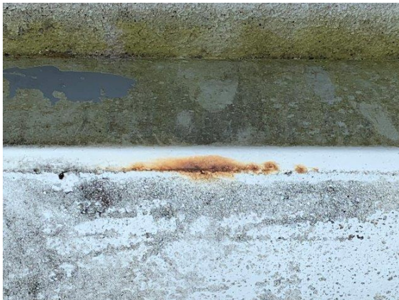
Photo Exhibit No. 26 Corrosion on metal stair component should be touched up.
